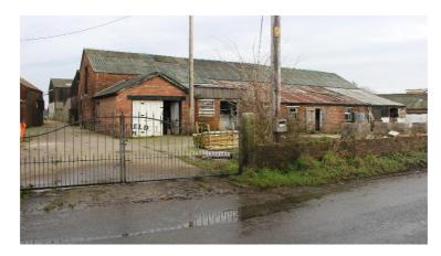
**Ex Parlour** (75' x 20') A mono pitch leanto building constructed from concrete block and red brick to part and a corrugated tin sheet roof. Internally the building has a concreted floor, concrete block stables.
