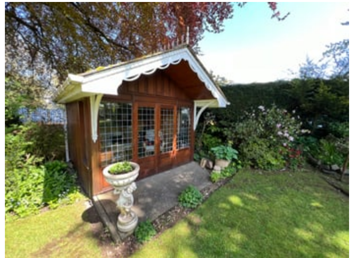
10' 0" x 9' 4" (3.05m x 2.84m) being of insulated timber construction with double glazed patio doors to front.
