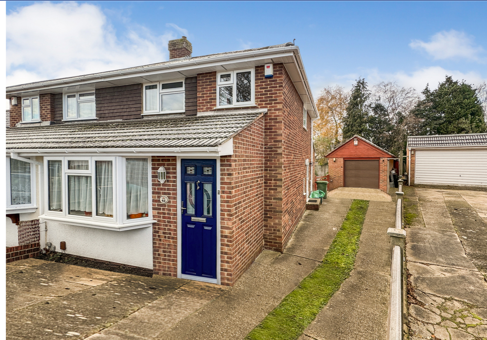
Skilton Road, Tilehurst, Reading.
