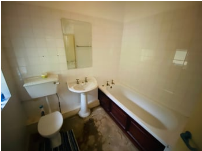
Having a fully tiled 3 piece suite comprising of panelled bath, low level flush w.c., pedestal wash hand basin, extractor fan.
