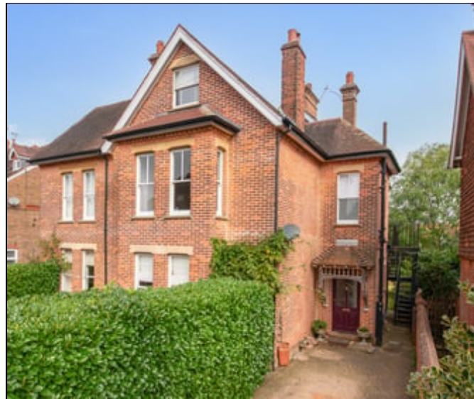
Covered porch to original front door.
