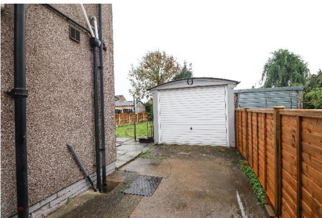
DRIVE LEADING TO GARAGE
