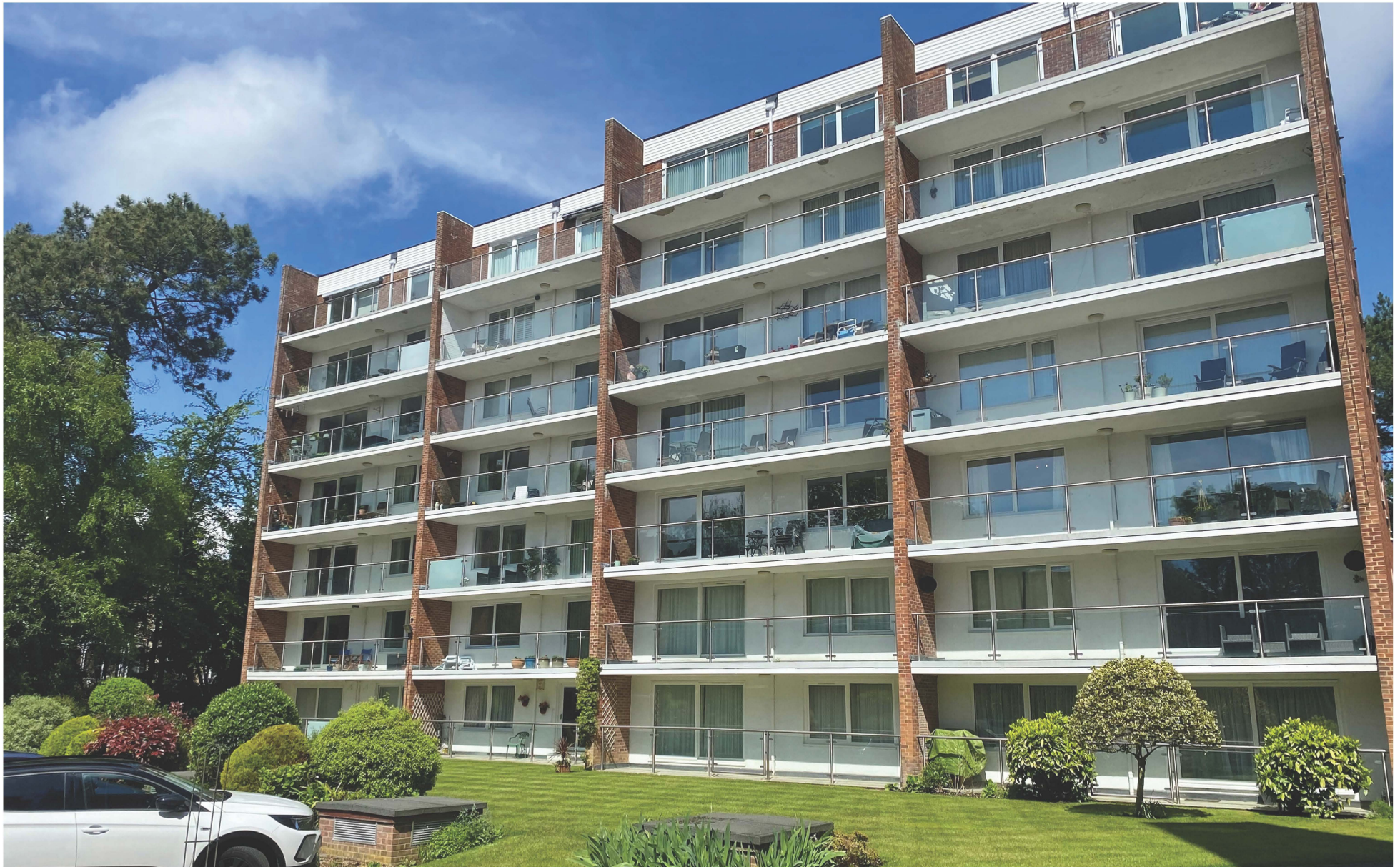
Sandbourne Road, Bournemouth BH4 8JP
