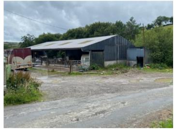
80' 0" x 43' 0" (24.38m x 13.11m). With separate overhang, feed barriers and concrete floor with clad roof and sides and block and shuttered walls.
