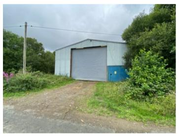
85' 0" x 45' 0" (25.91m x 13.72m). Formerly a Cattle shed with cubicles and loose housing facilities, of steel stanchion construction, clad roof and sides and wide doors for mechanical purposes.
