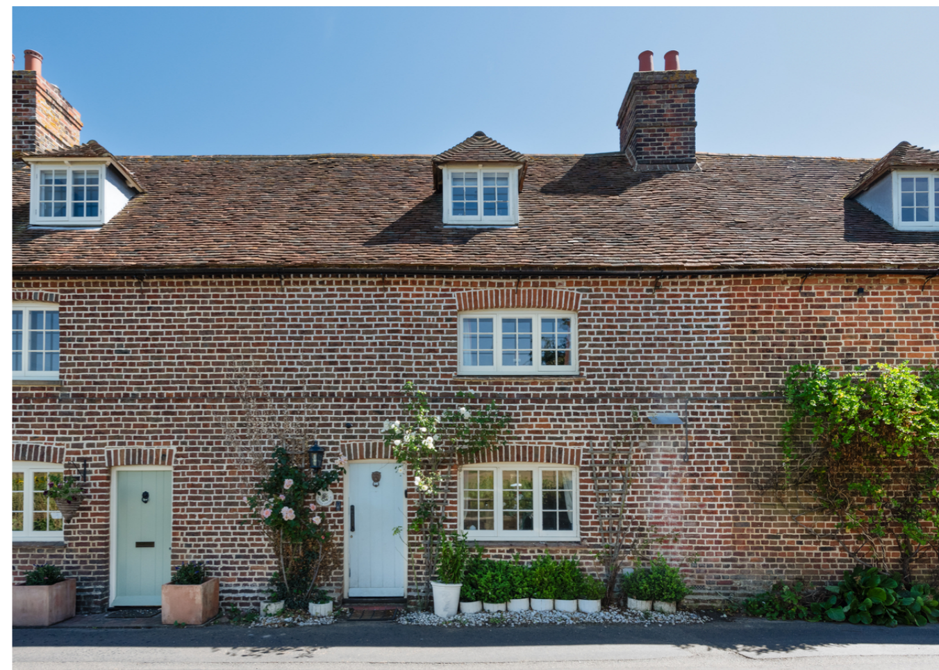
3 Middle Cottage, Hollow Street, Chislet, Kent, CT3 4DS
