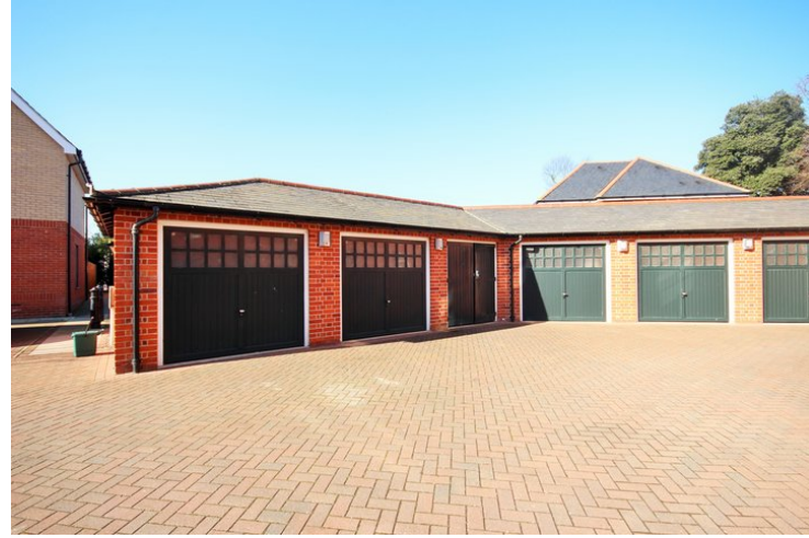
Timber garage doors.
