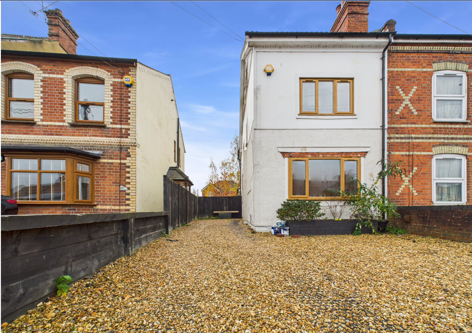
Norcot Road, Tilehurst, Reading, Berkshire. RG30
