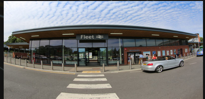
Fleet Mainline Railway Station
