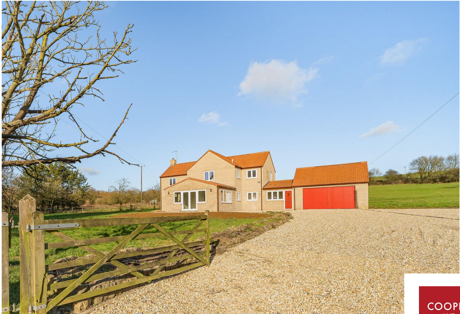
Manor Farmhouse, Prestleigh, Nr Shepton Mallet, BA4 4NJ
