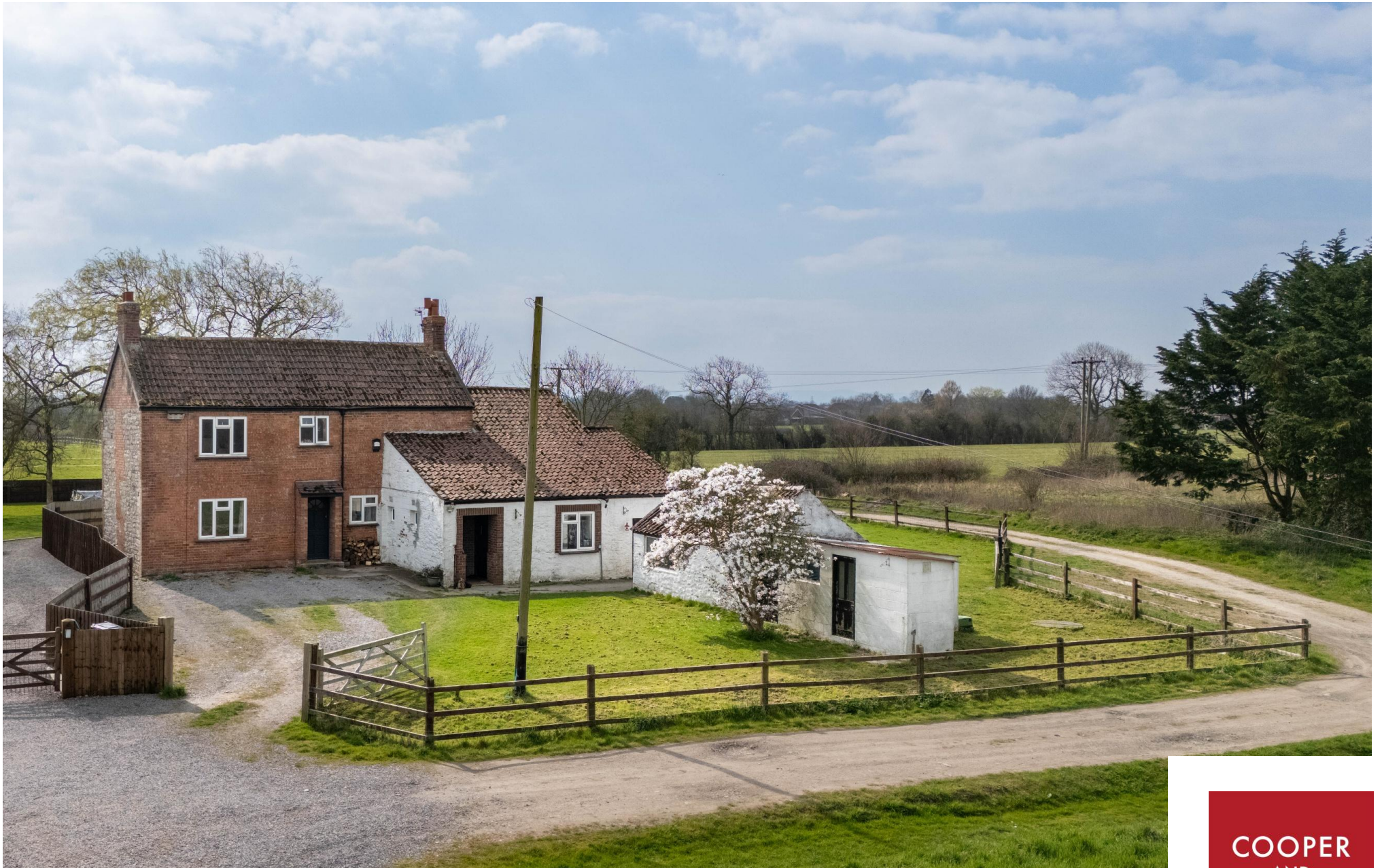
Moor Row Farm, Merry Lane, East Huntspill, TA9 3PS
