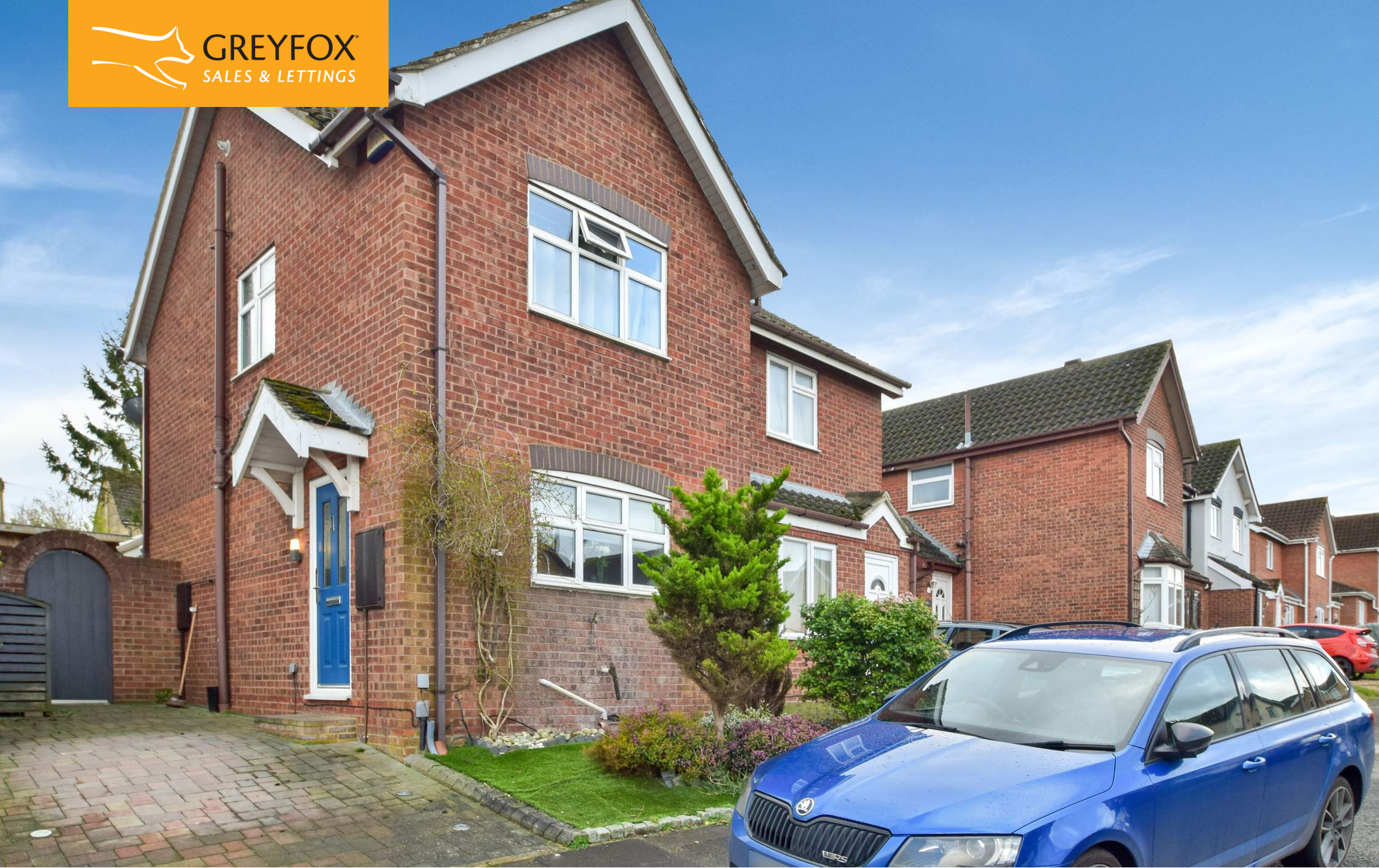
Two Bedroom Semi-Detached House Woolwich Close, Chatham, Kent, ME5 0HU
