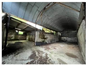
7' 5" x 16' 3" (2.26m x 4.95m) access doors to front and high level doors to rear, curved Dutch Barn style roof, concrete base.
