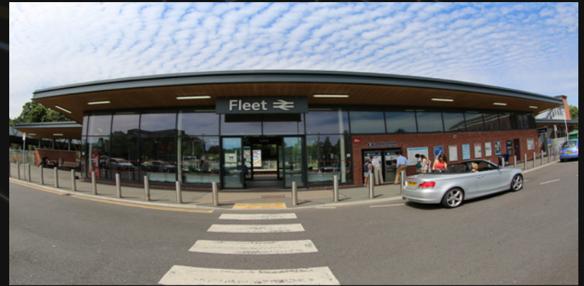
Fleet Mainline Railway Station
