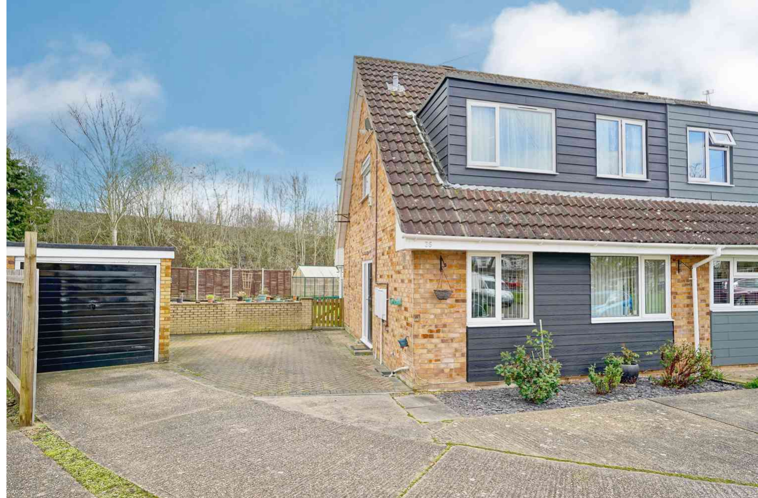
Manor Lane, Alconbury PE28 4EH
