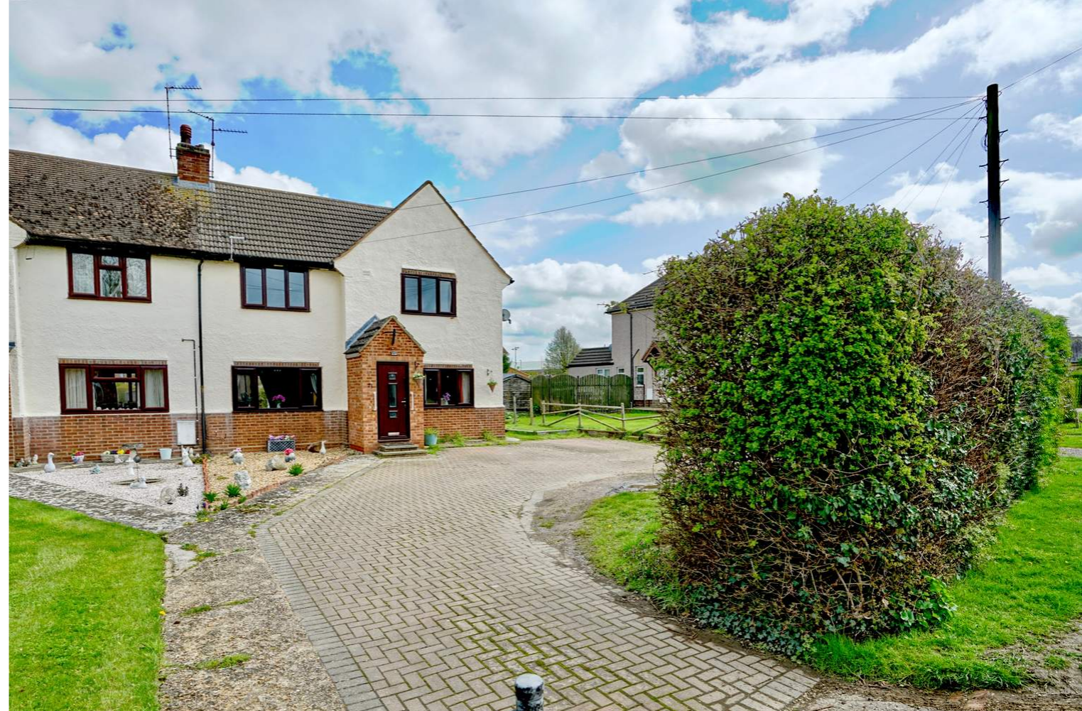
Green End Road, Sawtry PE28 5UX
