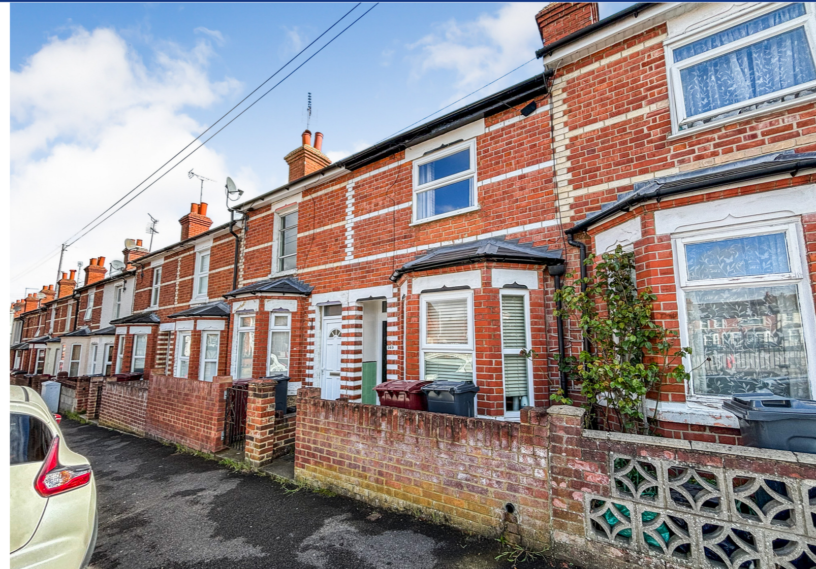
Cranbury Road, Reading, Berkshire.
