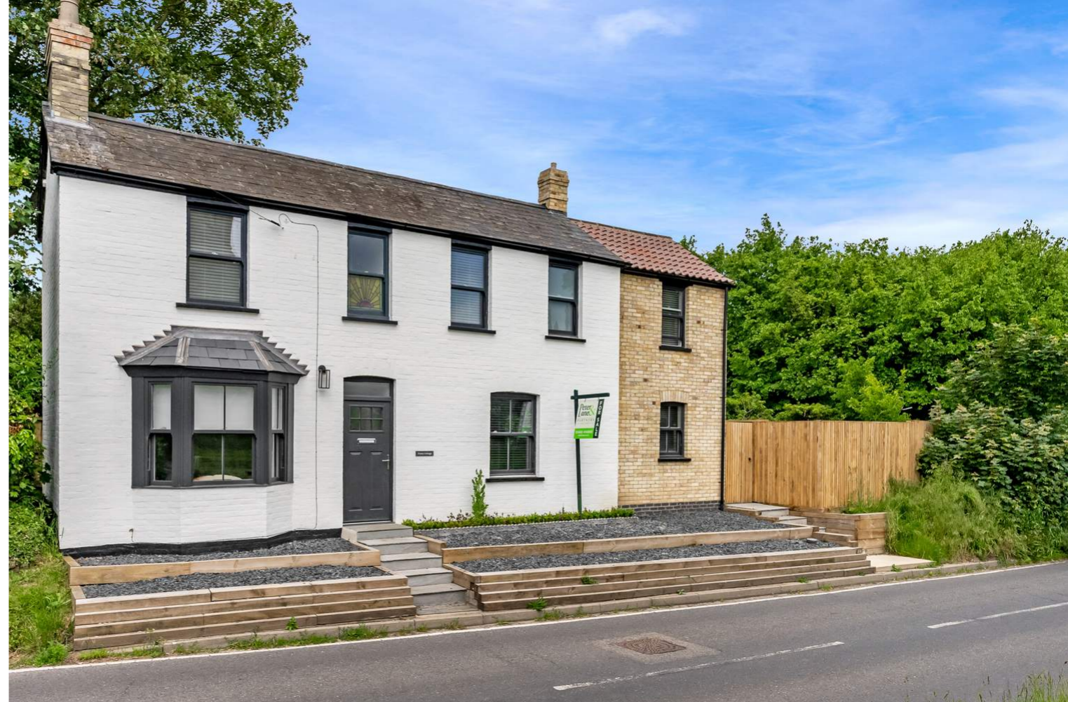
Ramsey Road, Kings Ripton PE28 2NJ
