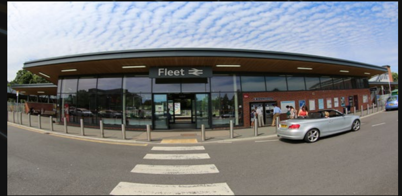
Fleet Mainline Railway Station
