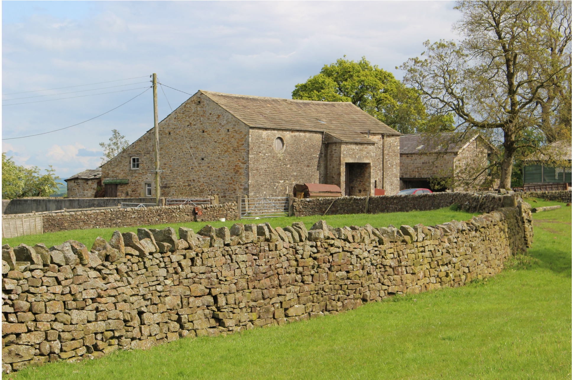
Four Bay Barn
