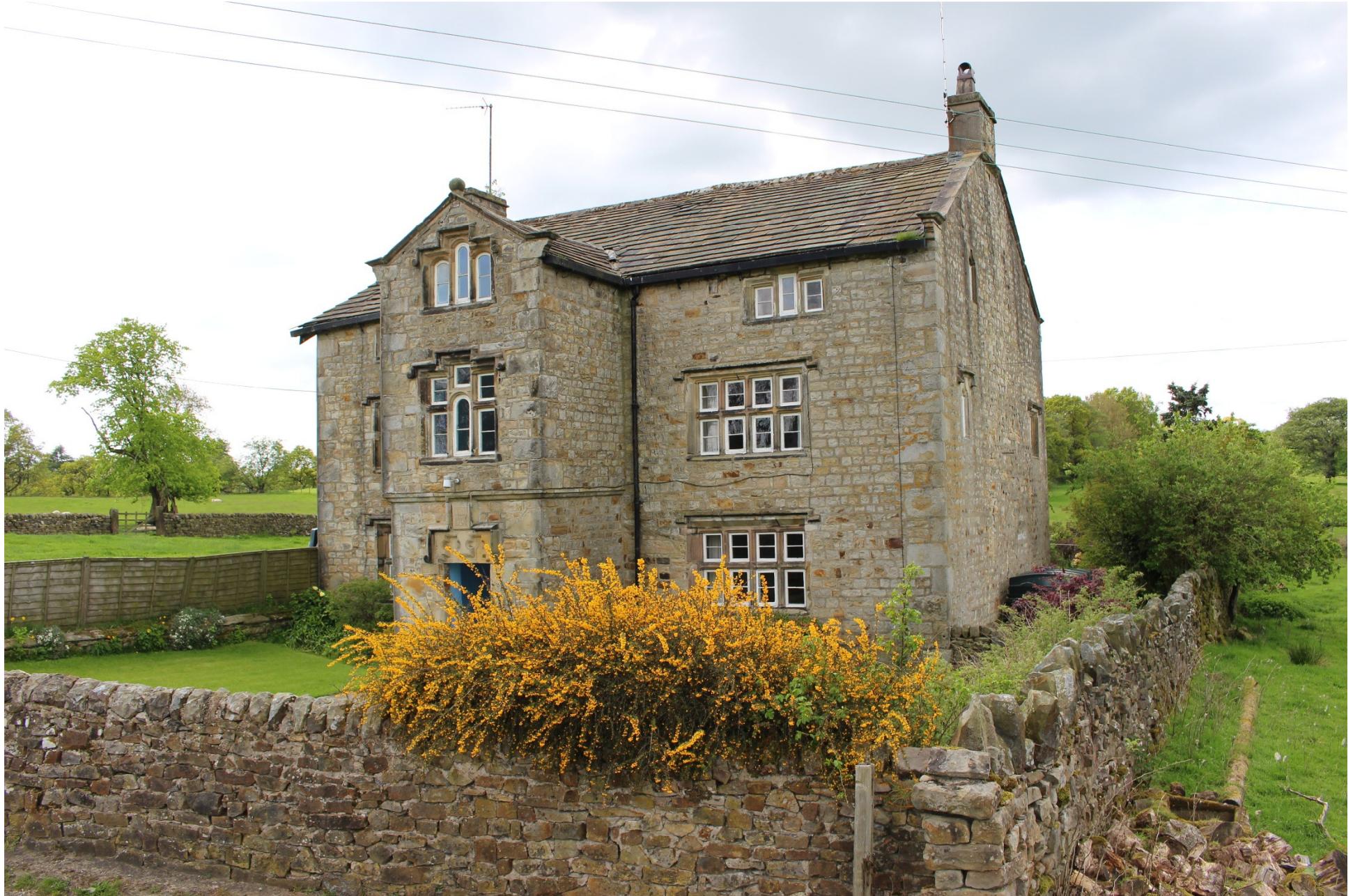
Grade II* Detached Residence
