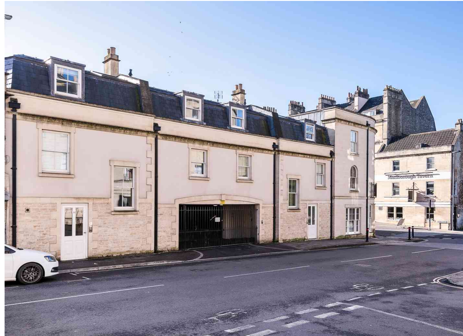
Crescent Lane, Bath
