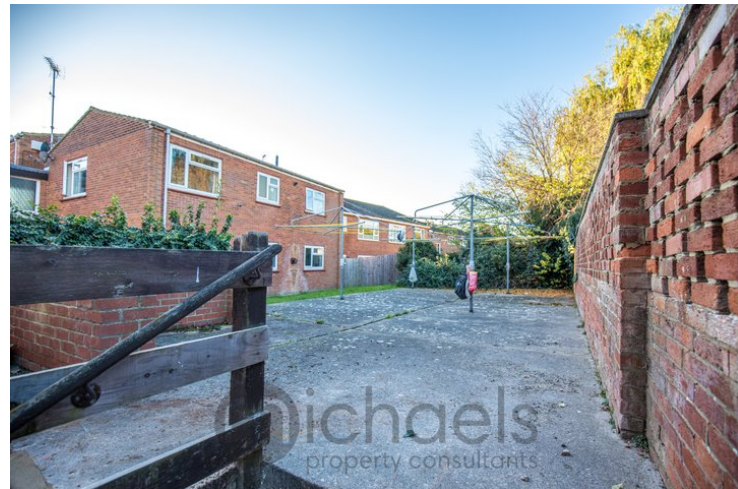
The block of apartments also resides within communal grounds and gardens, with ample parking available on a first come, first serve basis.
