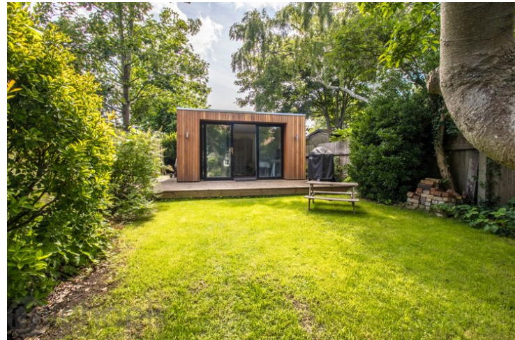
13' 5" x 10' 7" (4.09m x 3.23m) An excellent addition to the property, featuring glazed doors, light and power. Making the ideal work from home space, gymnasium or outdoor snug area.
