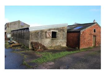
**Shippon** (65' x 14') (Building No. 2 on site plan) A monopitch ex cow shippon with corrugated tin roof sheets to the roof and sides, concrete floor in a dilapidated condition.
