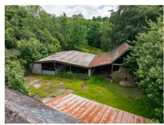
$60'\ 0"\ x\ 40'\ 0"$  (18.29m x 12.19m) steel framed and open fronted, previously used for livestock loose housing and feed passage.
