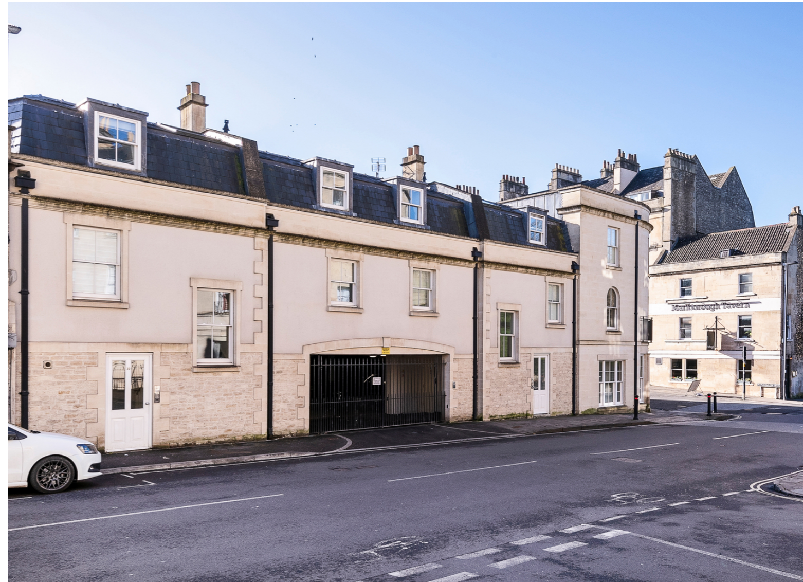
Crescent Lane, Bath
