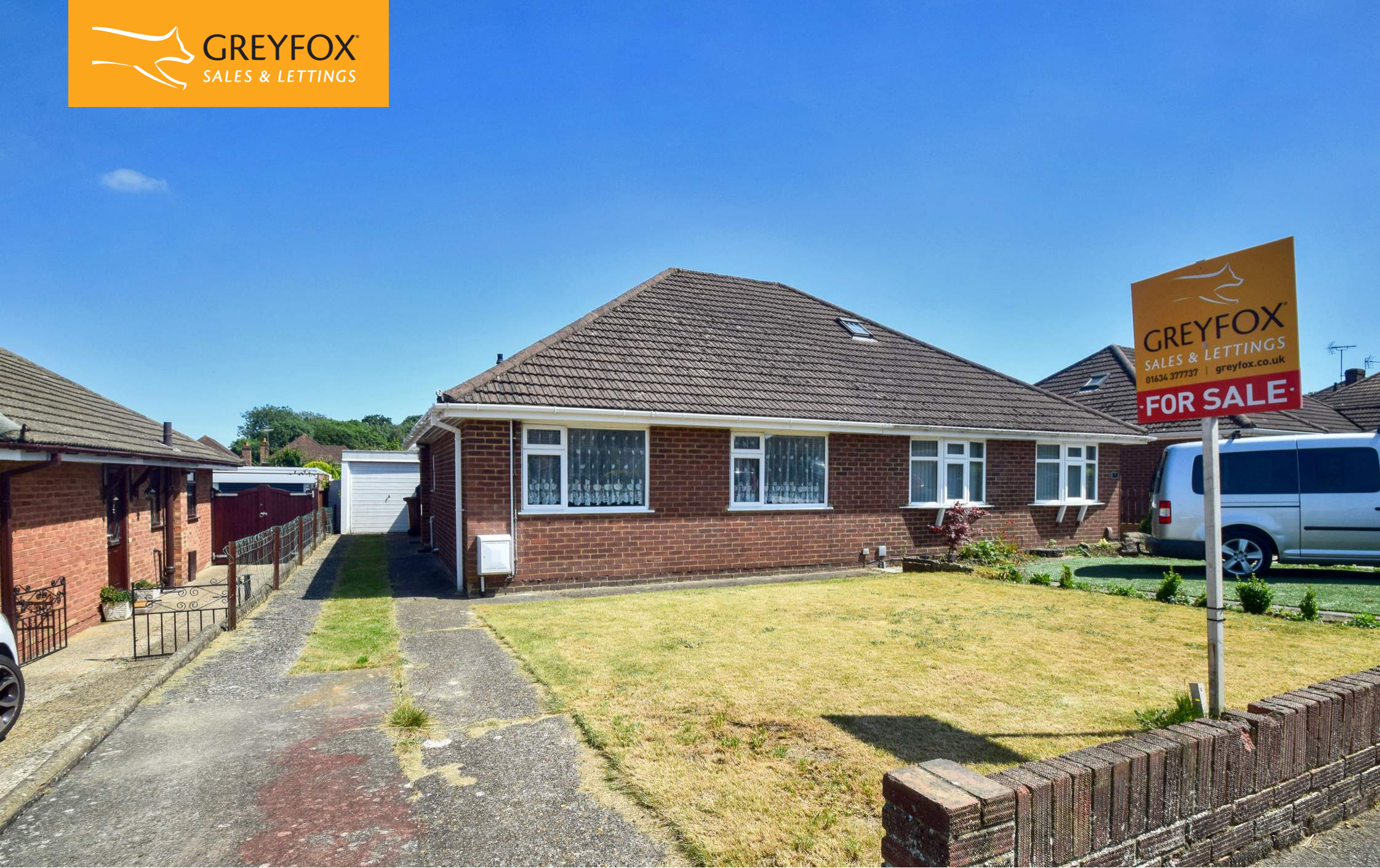
Two Bedroom Semi-Detached Bungalow St Margarets Drive, Wigmore, Gillingham, Kent, ME8 0NR
