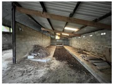
75' 0" x 21' 0" (22.86m x 6.40m) with rear access door, concrete base, a modern steel frame building of steel frame construction with a box profile cladding to walls and roof. 30' high open access to front, split into 3 separate sections.
