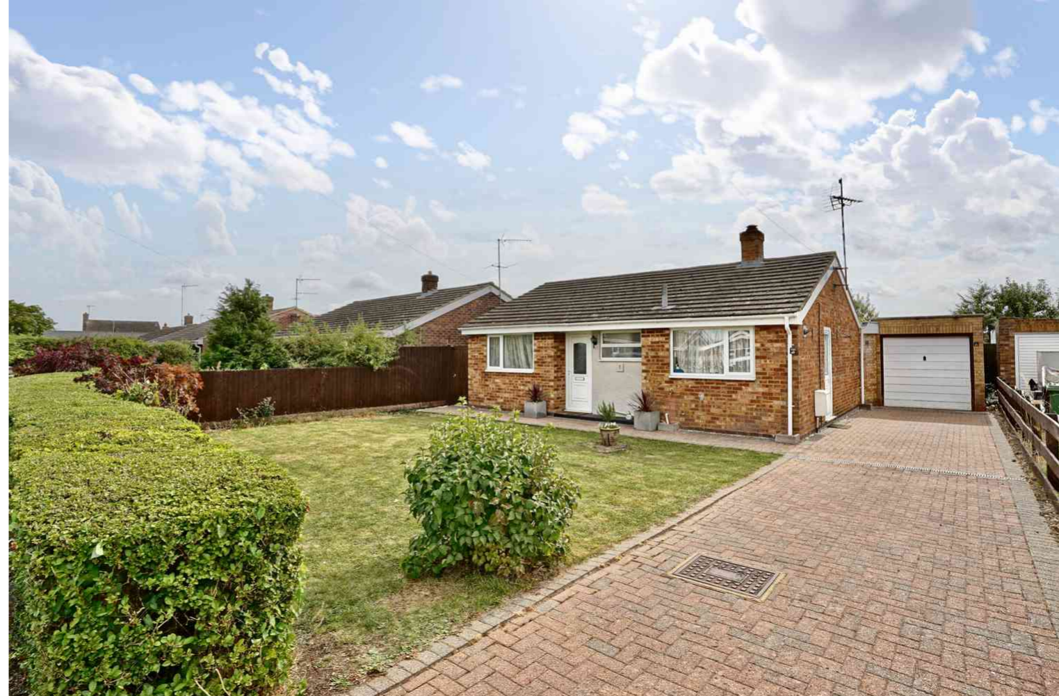
Aversley Road, Sawtry PE28 5XD
