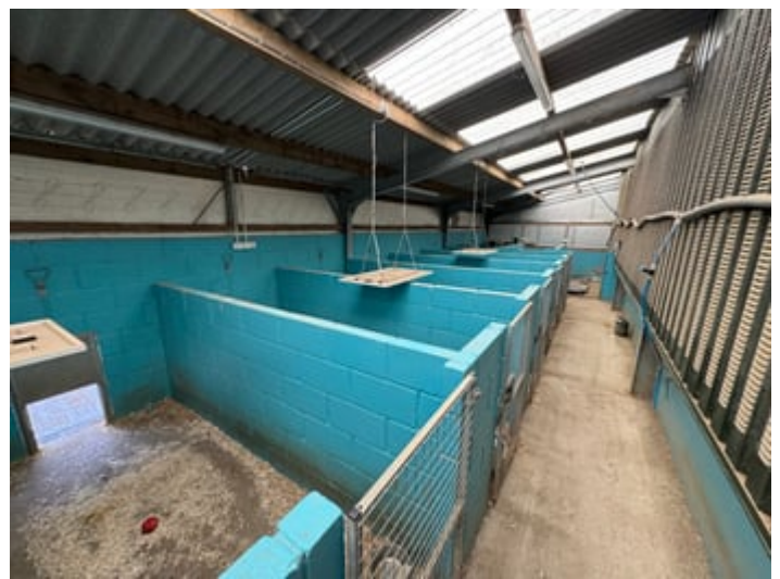
15' 0" x 60' 0" (4.57m x 18.29m) of steel frame with block and box profile walls providing 11 kennels and dog run areas with concrete base and water and electric connection.
