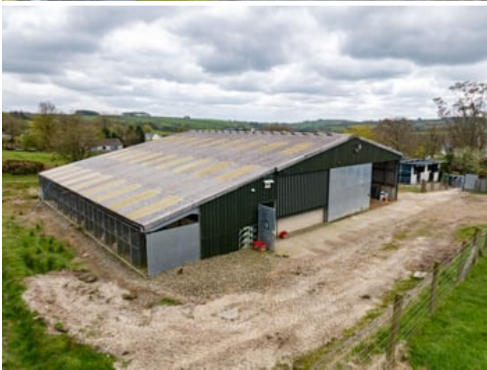
60' 0" x 45' 0" (18.29m x 13.72m) recently constructed with concrete shutter panelling and box profile panelling to walls, cement fibre roof, water and electric connection, 16' to ridge, sliding steel door to front.
