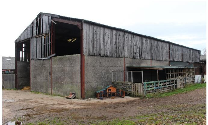
**Stable Block** (90' x 30') A steel portal frame building with concrete floor, concrete block walls and timber clad with a corrugated fibre cement roof. Internally the building is sectioned into 9 stables with a 2 stable leanto on the south elevation. All stables are concrete block with split stable door fronts.
