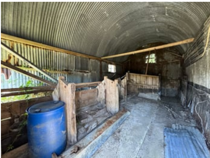
30' 0" x 15' 8" (9.14m x 4.78m) a former additional parlour and dairy with cow ties, timber frame and zinc clad construction with side lean-to, last used for storage.
