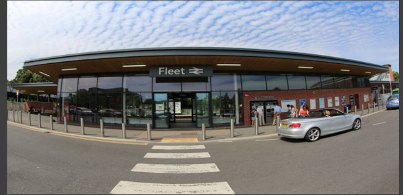
Fleet Mainline Railway Station
