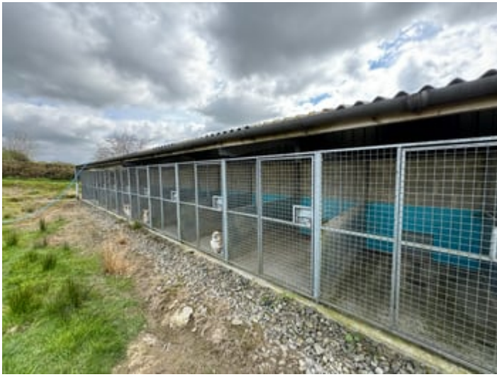
15' 0" x 60' 0" (4.57m x 18.29m) of steel frame with block and box profile walls providing 11 kennels and dog run areas with concrete base and water and electric connection.
