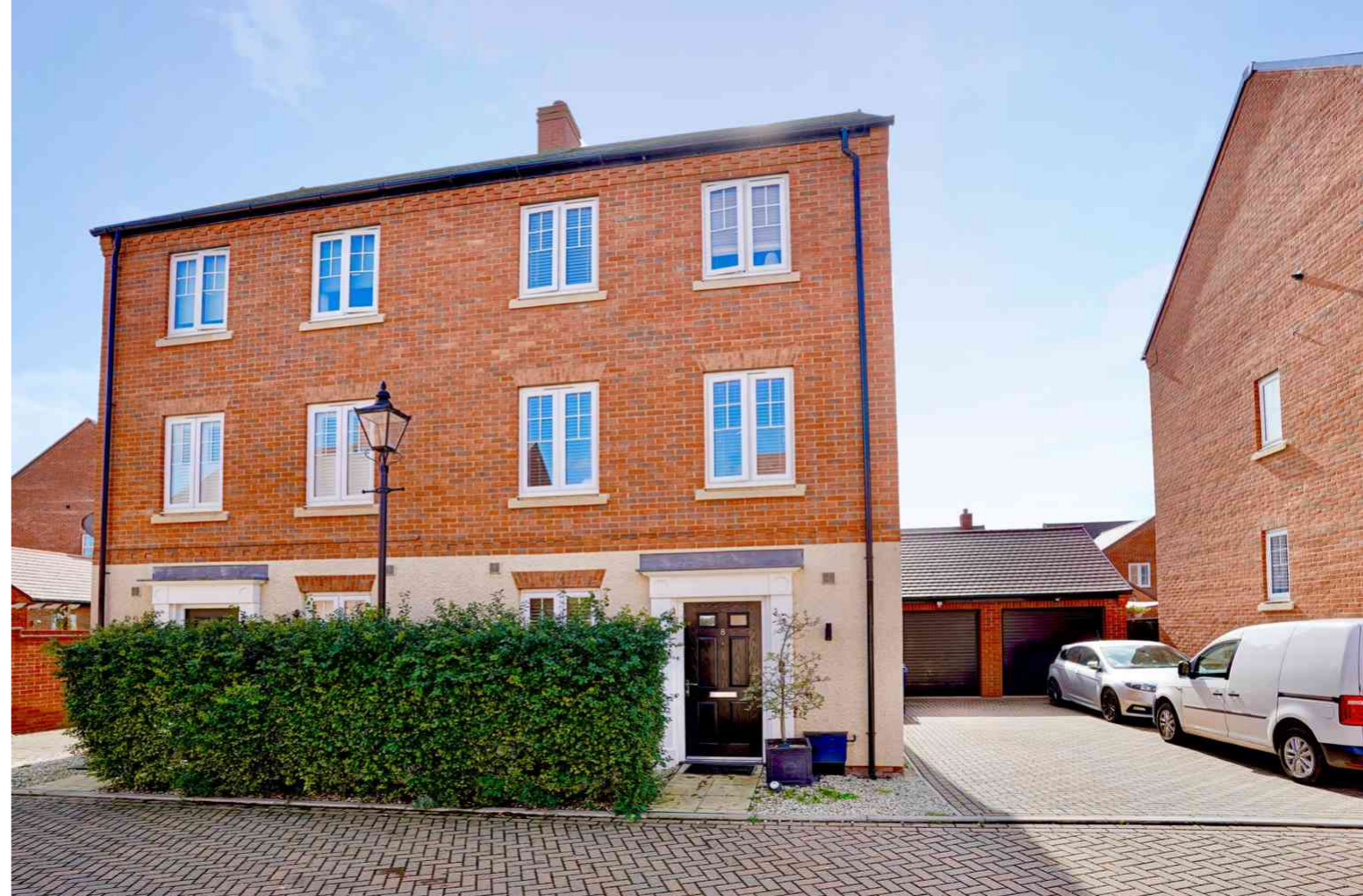
Griffin Road, Brampton PE28 4QP
