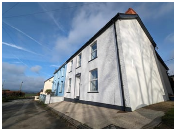
The property is approached from the adjoining county road to a concrete plinth with space for 2 vehicles to park. Side footpath leading through to -
