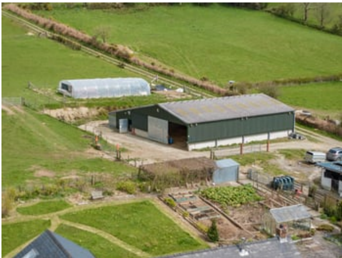
60' 0" x 45' 0" (18.29m x 13.72m) recently constructed with concrete shutter panelling and box profile panelling to walls, cement fibre roof, water and electric connection, 16' to ridge, sliding steel door to front.
