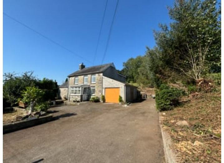
FRONT OF PROPERTY
