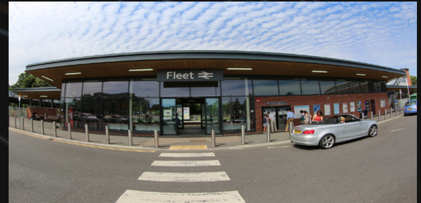
Fleet Mainline Railway Station
