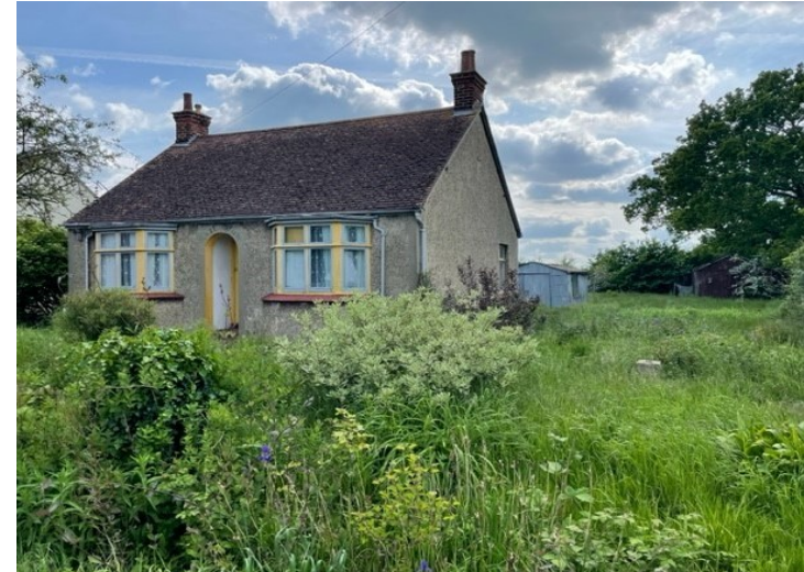
Front of Existing Property
