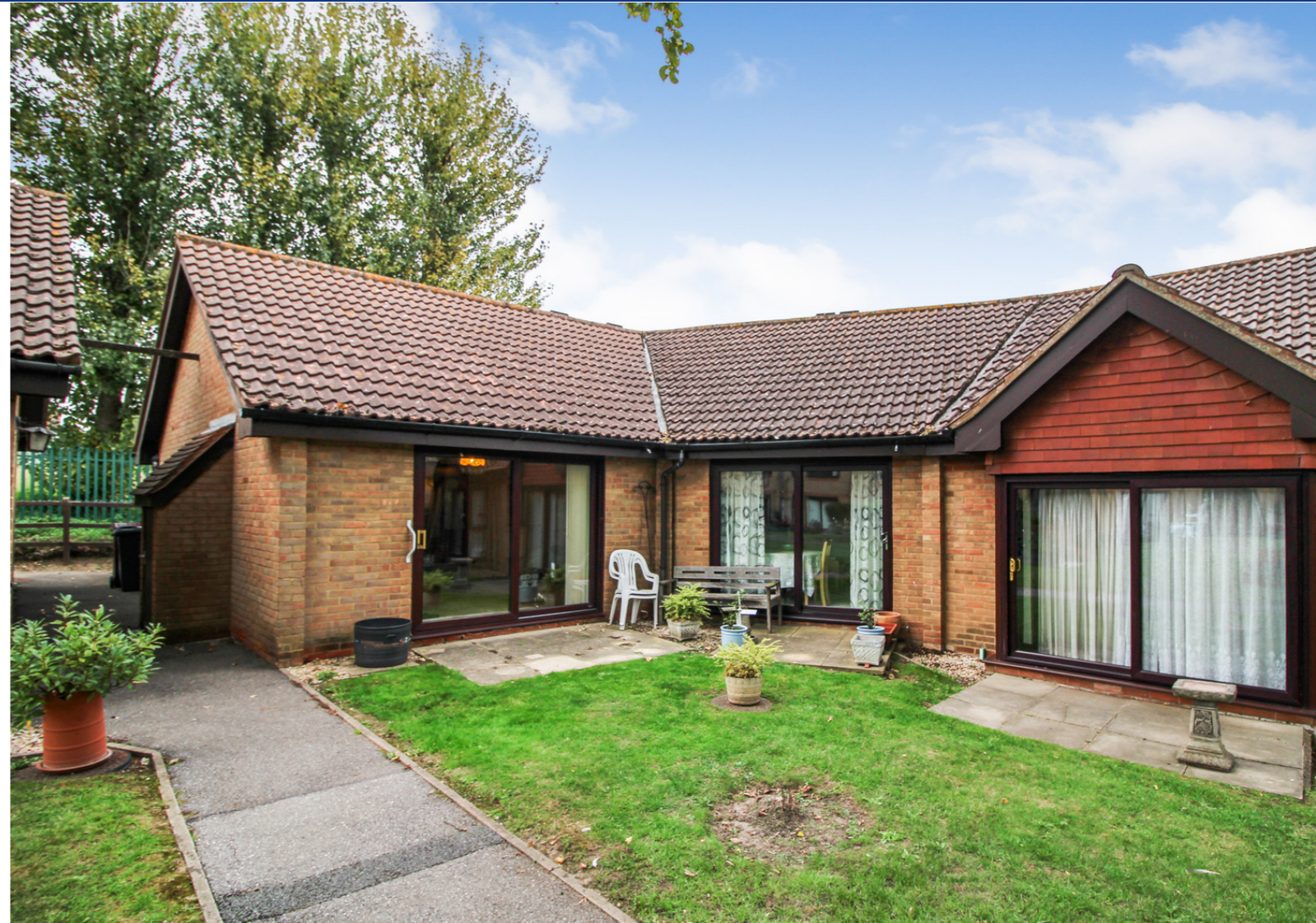
Burrcroft Court, Reading, Berkshire.
