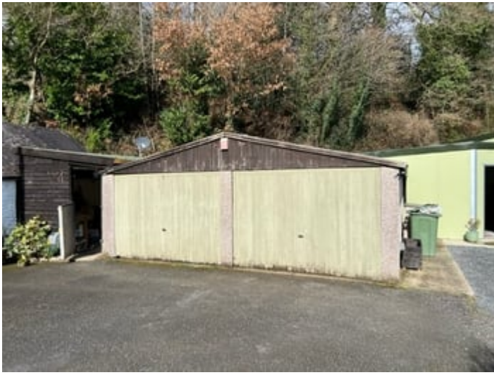
Covered Tractor/Log/Store Processing Building.
