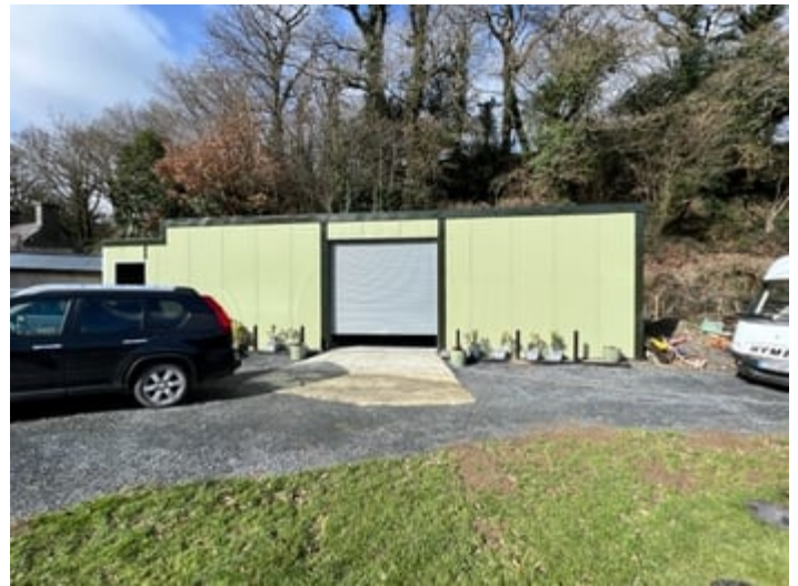
Adjacent Store Room
