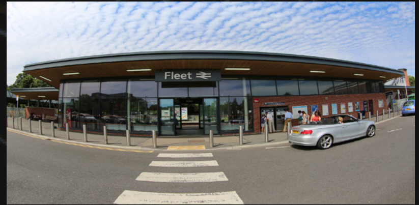
Fleet Mainline Railway Station
