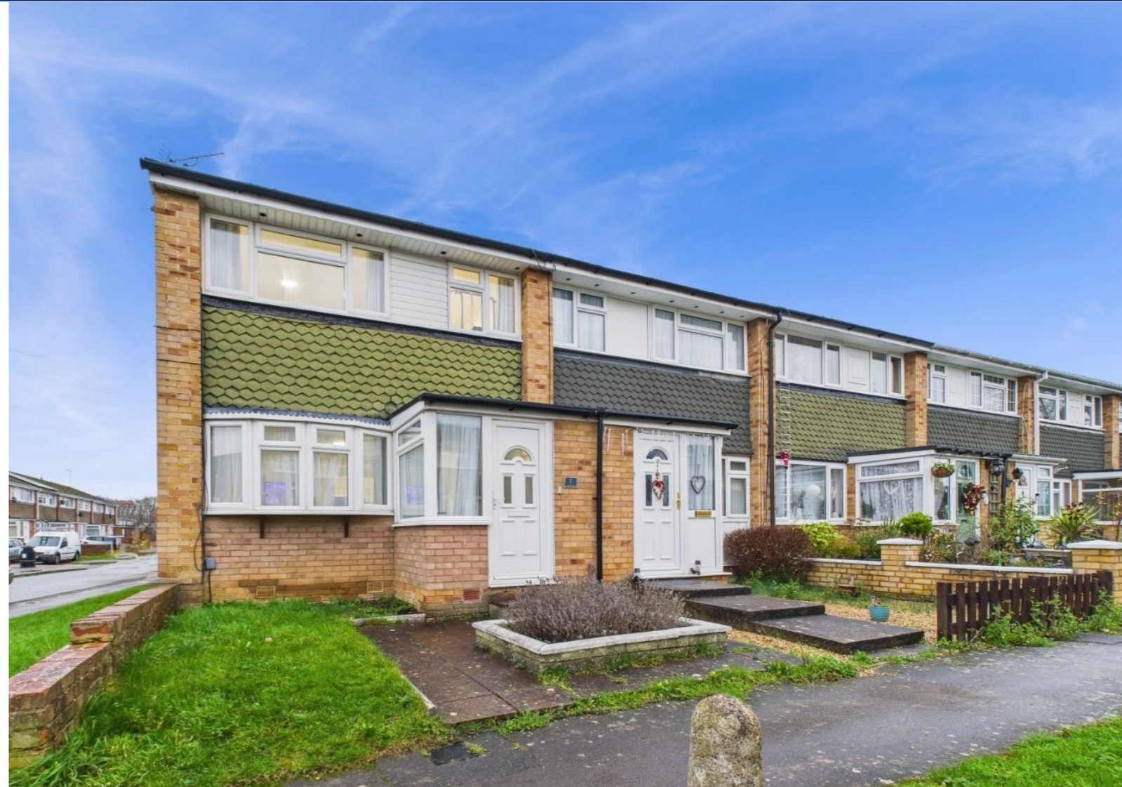
Poole Close, Tilehurst, Reading, Berkshire. RG30.
