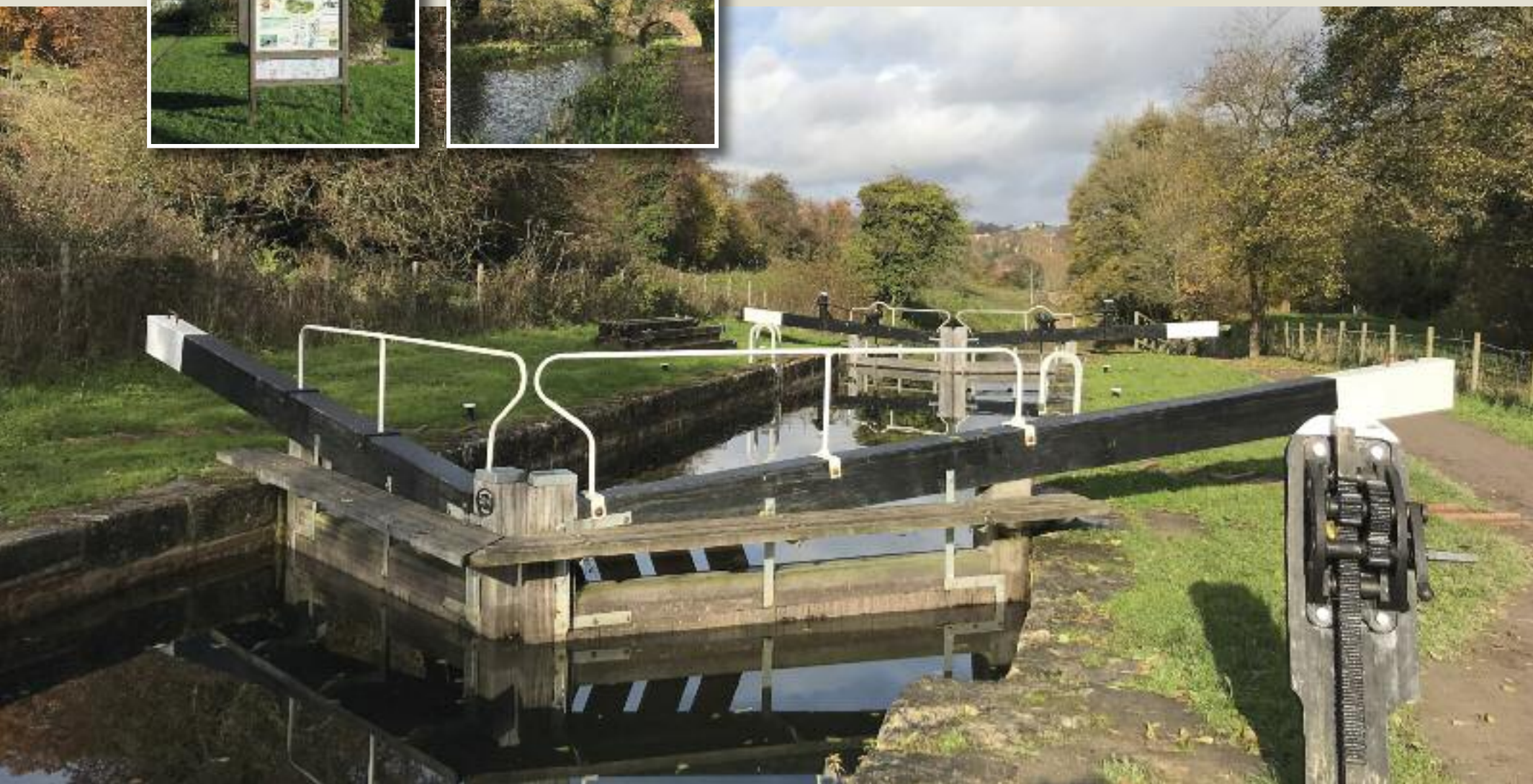
LOCK ON THE THAMES AND SEVERN CANAL, THRUPP
