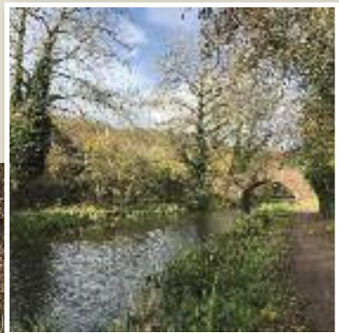
SEVERN AND THAMES CANAL, CHALFORD BAGPATH BRIDGE, SEVERN AND THAMES CANAL
