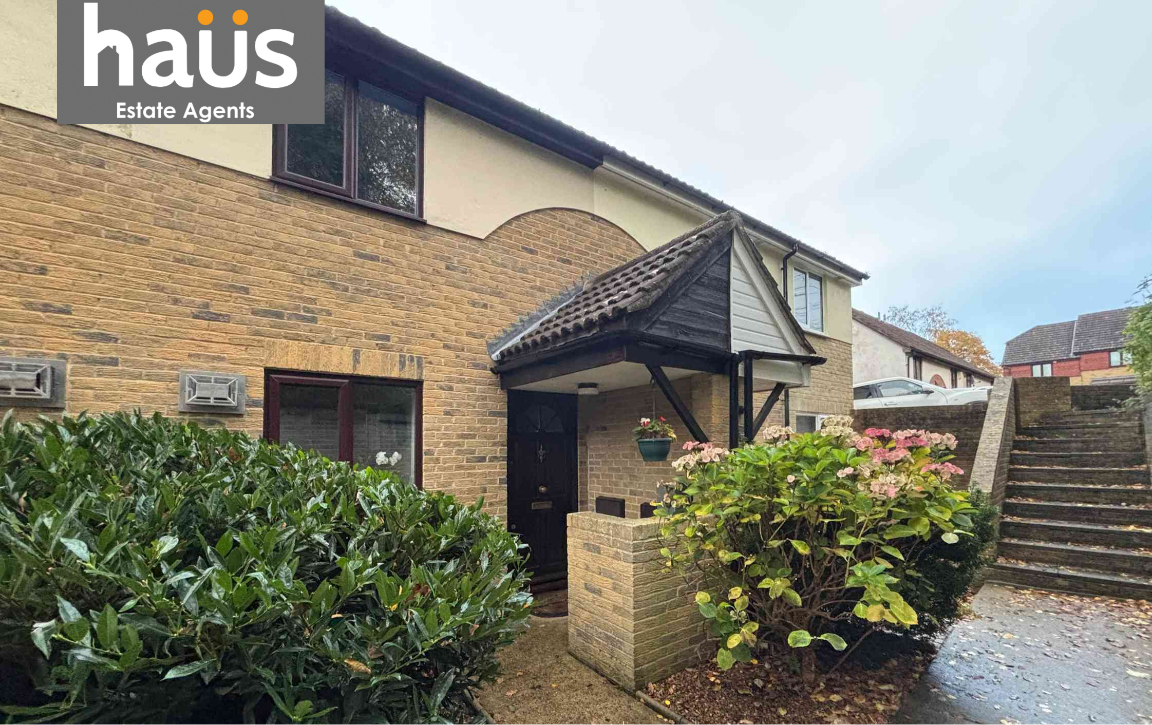
Two Bedroom Terraced House Alexandra Glen, Chatham, Kent, ME5 9EB
