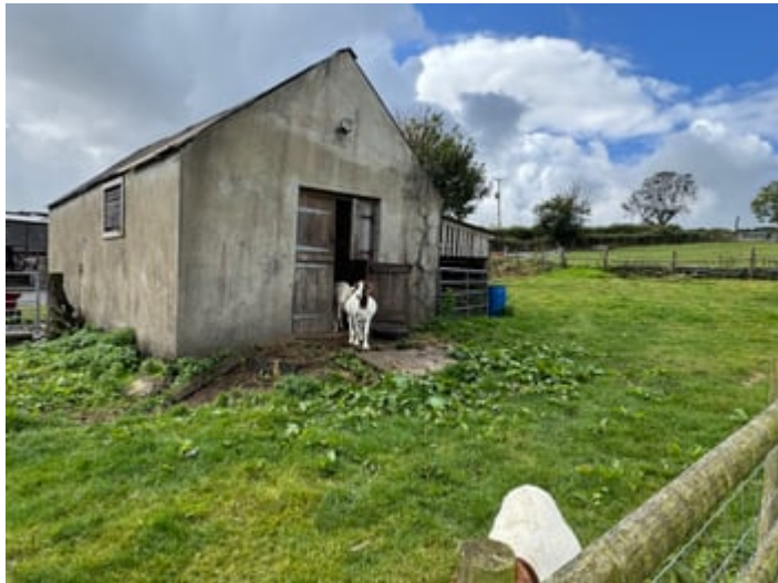
Concrete built and rendered stable building.
